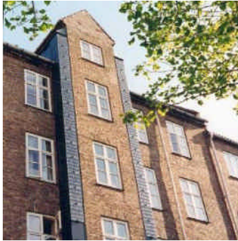
Fig. 2.9.2: PV-assisted solar ventilation towers and PV-chimney were PV modules are directly operating DC-fans.
