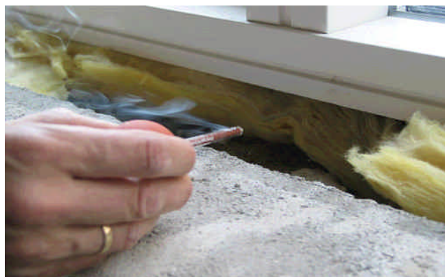
Fig. 2.3.2: Example of registration of white smoke movement to trace cracks and crevices in combination with the blower door test.
