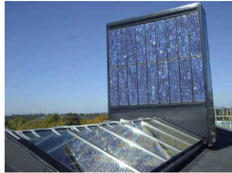
Fig. 2.9.2: PV-assisted solar ventilation towers and PV-chimney were PV modules are directly operating DC-fans.
