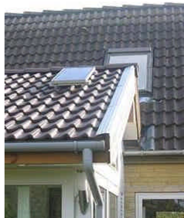
Fig. 2.9.1: Small ventilation unit for sunspaces which is operated by help of a small PV-plant, which produces the needed electricity for operation of the fan. A operation the fan. A ventilation rate up to 400 m 3 /h is possible. FK: The PV module is about ¼ m 2 , so it generates about 25Wpeak, which is far too little to drive the heat pump.
