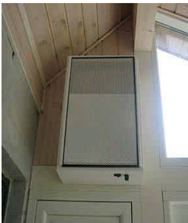
Fig. 2.9.1: Small ventilation unit for sunspaces which is operated by help of a small PV-plant, which produces the needed electricity for operation of the fan. A operation the fan. A ventilation rate up to 400 m 3 /h is possible. FK: The PV module is about ¼ m 2 , so it generates about 25Wpeak, which is far too little to drive the heat pump.
